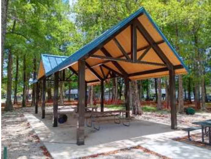
The new, larger pavilion at Veterans Park will replace two smaller ones and be available for events
