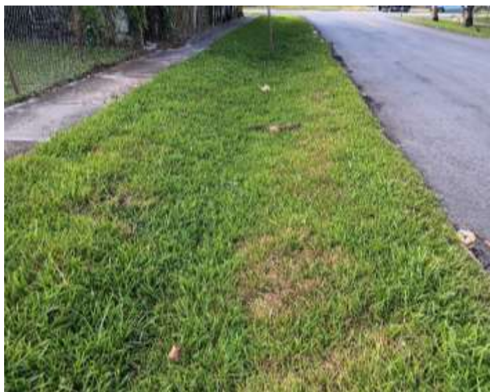
Completed swale on NW 17 Court after work by Weekley Construction to lower and re-sod
