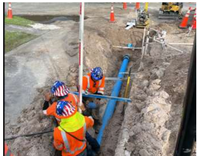
Replacement of water lines on Lime Hill Road has been completed. NW 82 Ave will be the next water line upgrade.
