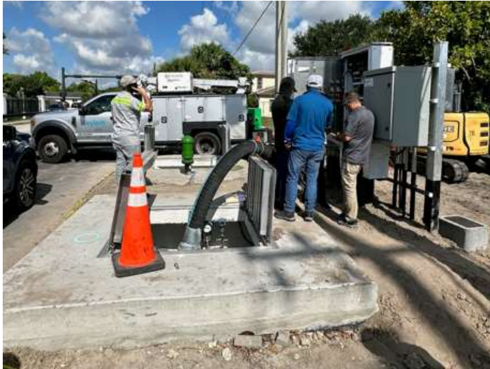
Lift station # 15 being tested prior to starting operations. Final phase is restoration of curbing and sidewalks.
